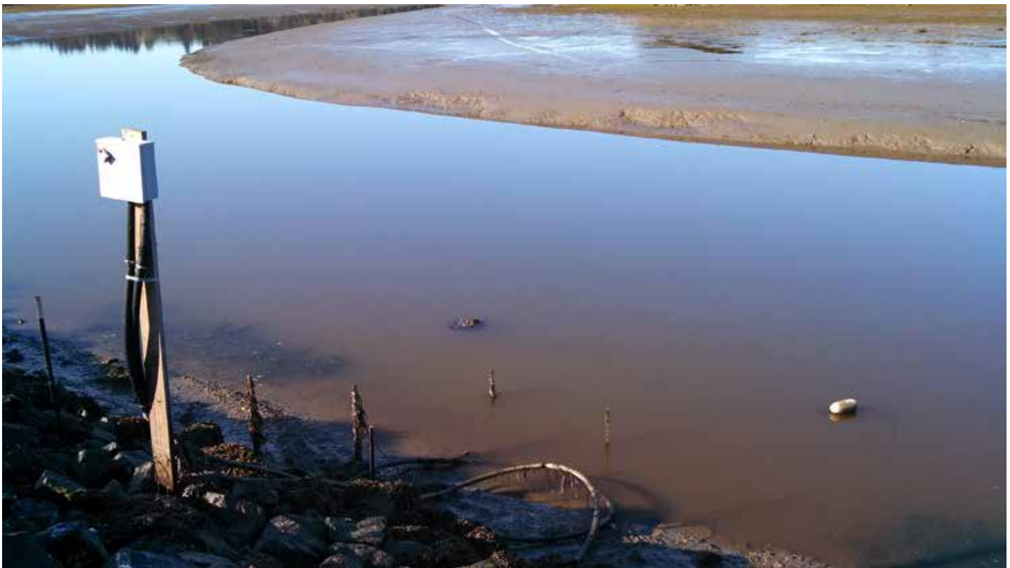
Figure 4. A. Location Map Hookton Slough Tide Gage. B. Tide gage installation site photo.
